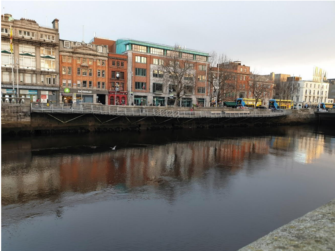
Existing footbridge similar to Ringsend 02 upstream the proposed site – Looking from south river bank
